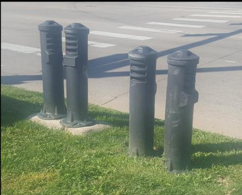
Blue Water Innovations, LLC has developed an innovative street vent assembly that is light weight and durable. With it's patented quick change air flow vent cap and 150psi flange bolt hole pattern base, this system was designed to improve operational efficiencies and installation time.
